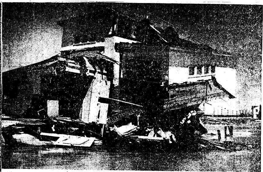
The Potter home on Dune Road, Westhampton Beach—house was turned 45 degrees by tide.
