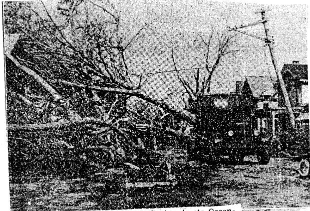
15. Main and Center streets, Greenport.
