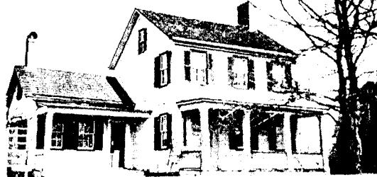
THE FIRST HOUSE Andrew Gildersleeve built (in 1839) now has the Red Barn antique shop in its barn. Left, in its earlier days; right, as it will be pictured in the New York State files.
